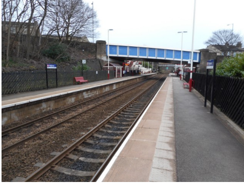
The Station in Early 2015
